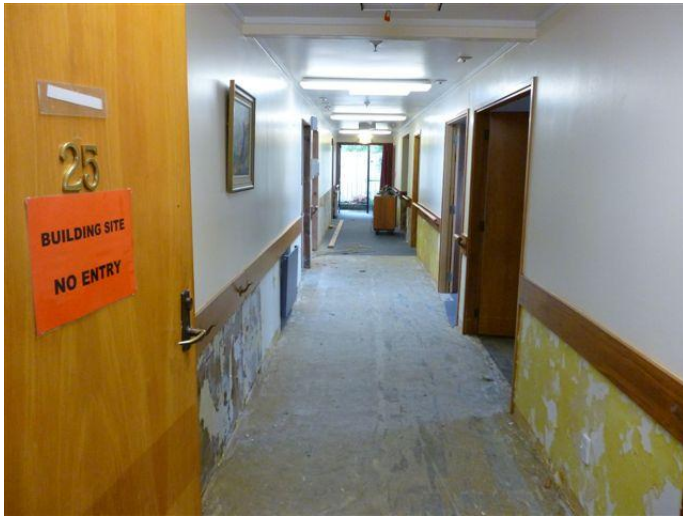
Hospital wing corridor
